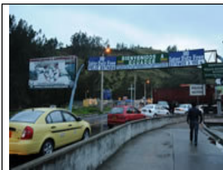
Rumichaca International Bridge, joining Ecuador and Colombia, is in Carchi; this is where Colombians fleeing from the violence of the internal conflict in Colombia enter the country. UNHCR/M. Fernández
